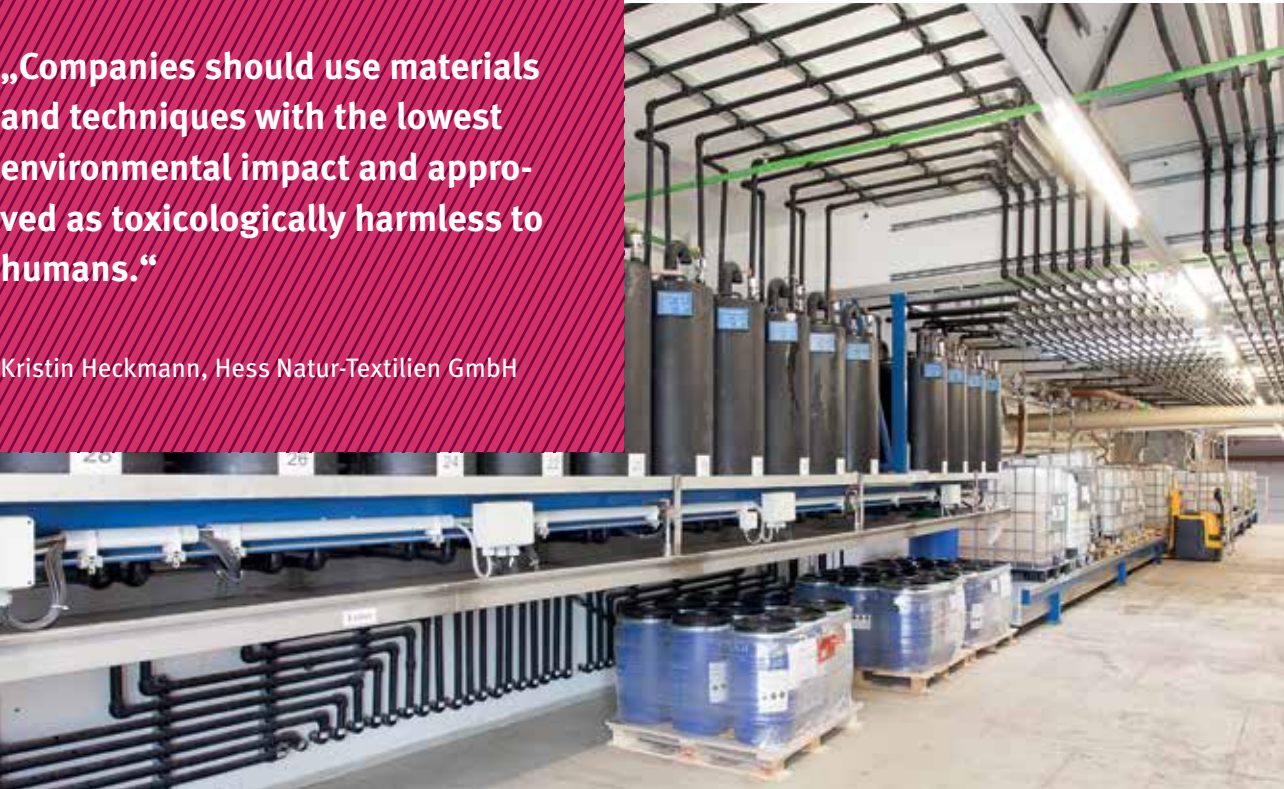
Optimized transfer of chemicals from storage to the batching tanks. The tanks are directly connected with the chassis.
